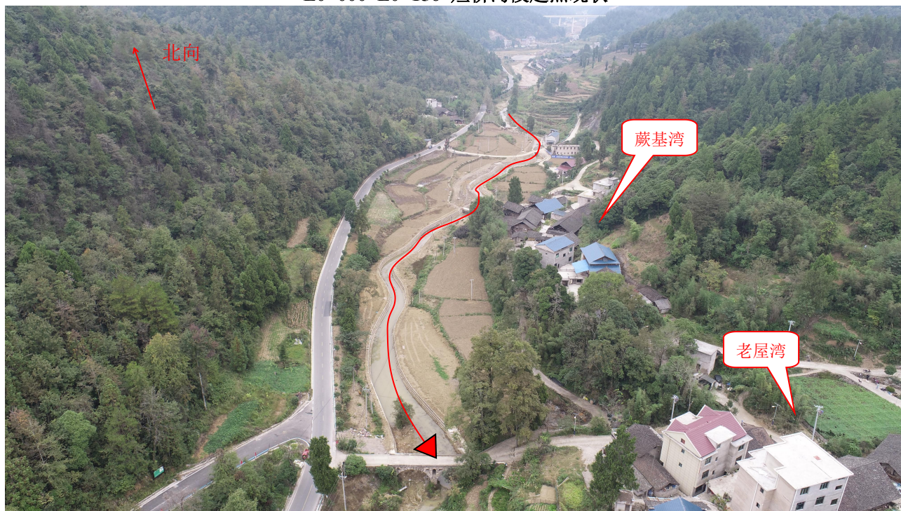
YA5+260~YA5+733 异溪沟主干段现状
